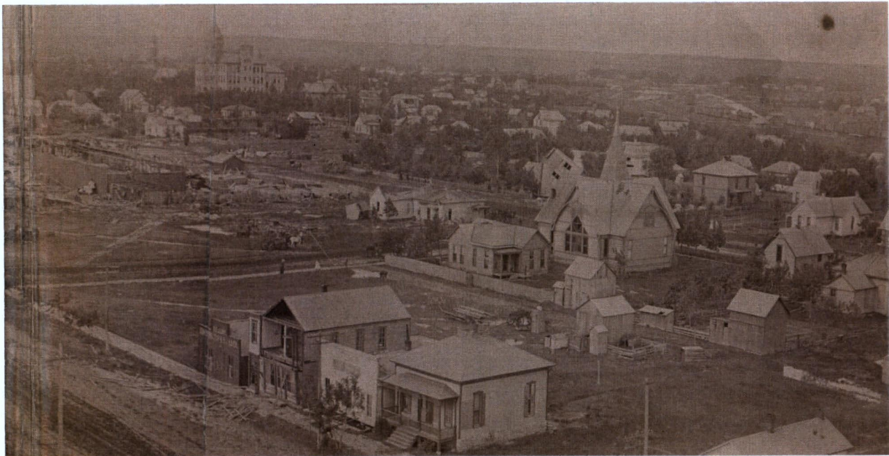
1893 Wellington Tornado damage—donated by the City of Wellington
