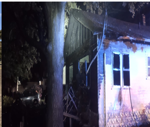
Structure Fire 1200 block North A
