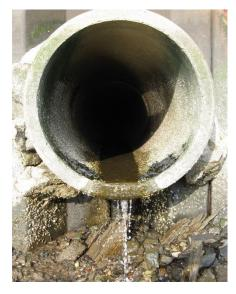
Many of the existing sanitary sewer pipes in the downtown area are older clay pipes. Clay pipes of this age may have deficiencies leading to inefficiencies and potential sewage back-ups. It is recommended that the pipes be inspected to identify any deficiencies and necessary improvements. Based on discussions with City staff, there are not any known capacity issues in the system.
